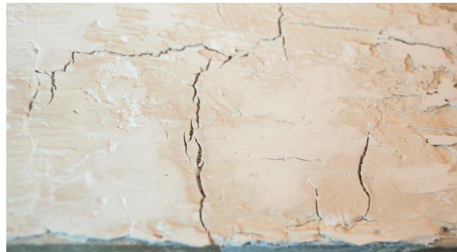
Figure 21: B-72 before sanding showing deep cracks in surface
